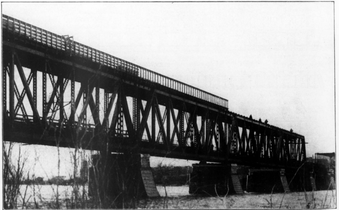
FIG. 6. NEW DOUBLE-DECK SPANS OF THE KEOKUK BRIDGE
