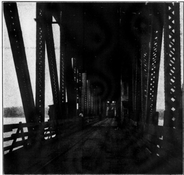
The New Draw Span with the Old Highway Floor Still in Place
